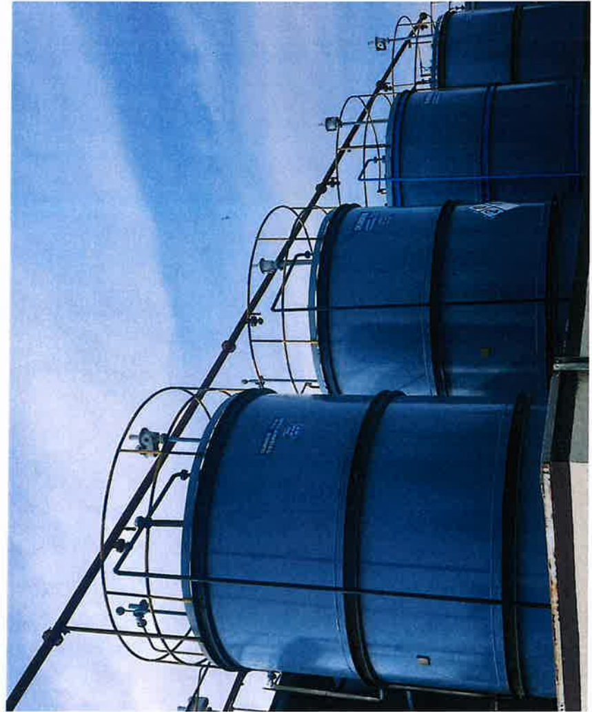
Provided breather valves along with nitrogen blanketing system for all the solvent storage/chemical storage tanks.
