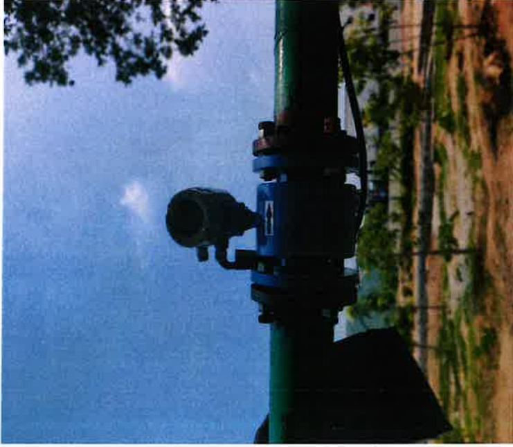
First runoff of rainwater collection tank with 300 KL & digital flow meter
