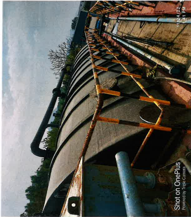
HTDS Dome with suction hood followed by two stage scrubbing system
